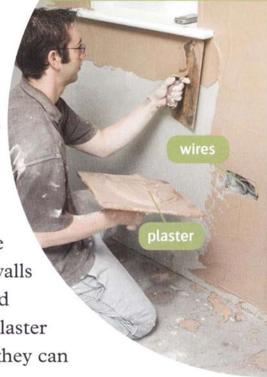
Putting Plaster on a Wall
