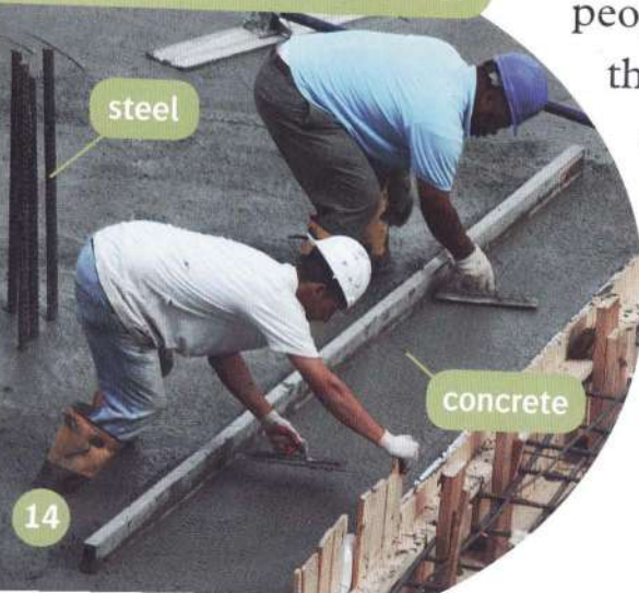
Making a Concrete Floor
